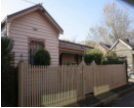
RICHMOND SHAMROCK STREET 5.jpg
