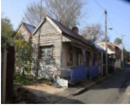
RICHMOND SHAMROCK STREET 7.jpg
