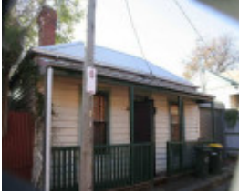
RICHMOND SHAMROCK STREET 9.jpg
