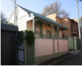
RICHMOND SHAMROCK STREET 11.jpg
