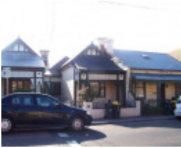
RICHMOND BAKER STREET 55.jpg
