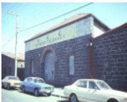
former melvilles grainstore colebrook street brunswick entrance
