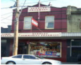
RICHMOND BURNLEY STREET 394.jpg
