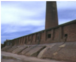
former hoffman brickworks dawson street brunswick side view & chimney
