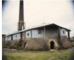
former hoffman brickworks dawson street brunswick front view
