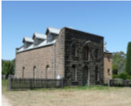
FORMER COBB & CO STAGING STABLES SOHE 2008
