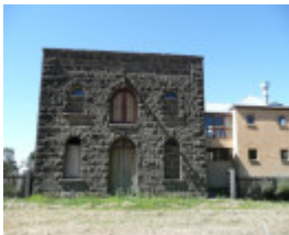
FORMER COBB & CO STAGING STABLES SOHE 2008
