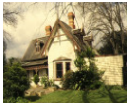
1 former curator's cottage queens park moonee ponds front view oct1994
