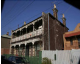
Richmond LESNEY STREET 20.jpg
