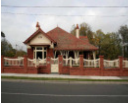
ALPHINGTON LUCERNE CRESCENT 2.jpg
