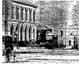
Ballarat Post Office02 - Colonnade enclosed, central entry maintained -Ballarat Conservation Study, 1978
