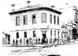
ANZ Bank02 - North west corner of Lydiard and Sturt Streets, showing the earlier bank building on the site - Ref: H26070 - La Trobe Library - Ballarat Conservation Study, 1978
