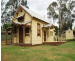
FORMER HEALESVILLE COURT HOUSE SOHE 2008
