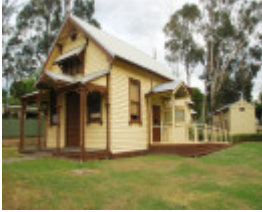
FORMER HEALESVILLE COURT HOUSE SOHE 2008
