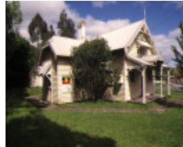
1 former healesville court house nicholson street healesville front corner view
