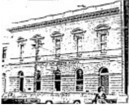
Bank of New South Wales - Film 1 / Frame 26 - Ballarat Conservation Study, 1978
