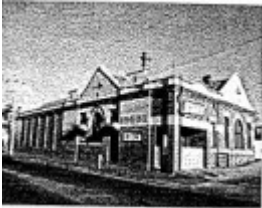
Offices Sunnyside Mills - Ballarat Heritage Review, 1998
