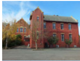
West elevation, Orphanage Additions (Building 5)
