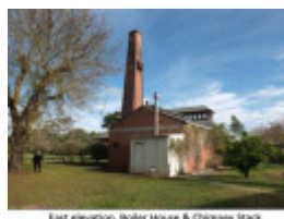
East elevation, Boiler House & Chimney Stack (Building 11)
