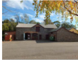
East elevation, Stables & Machinery Shed (Building 2)
