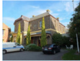
East and north elevations of Blythwood Garage (Building 1)
