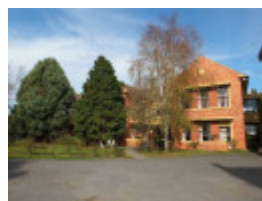
North elevation, Fatima House (Building 10)
