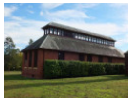
South & east elevations, former Laundry (Building 7)
