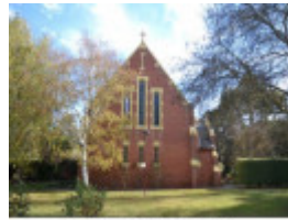
East elevation, Chapel (Building 4)
