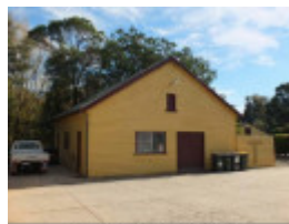
East elevation, Galined Shed (Building 8)
