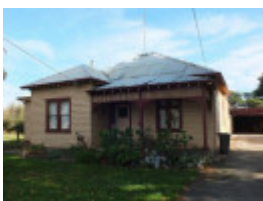
East elevation, former Caribaker's Dwelling (Building 9)
