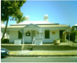
11 Villamanta Street, Geelong West
