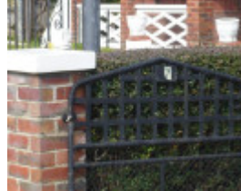
House and fence 7 Stanley Street
