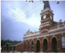
buninyong town hall street frontage dec1987
