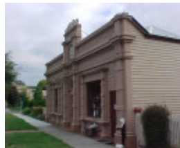
former library buninyong oblique front view 2002
