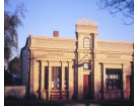
h00488 1 former library warrenheip road buninyong front view she project 2003
