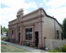
FORMER LIBRARY SOHE 2008
