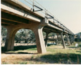
B3085 Janevale Bridge
