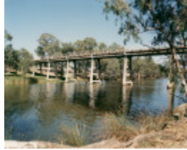
B3085 Janevale Bridge
