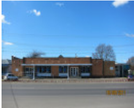
Sebastopol Town Hall complex - 1960 Borough Hall
