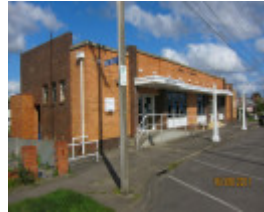
Sebastopol Town Hall complex - 1960 Borough Hall
