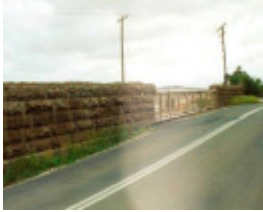
B7465 Riddells Creek Bridge
