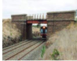
B7465 Riddells Creek Bridge
