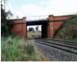
B7494 Forrest Road Bridge
