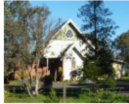
former St Francis Xavier Catholic Church, north elevation
