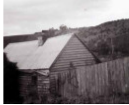
B3118 Outbuildings Caroline Chisholm Shelter
