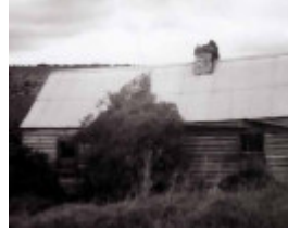
B3118 Outbuildings Caroline Chisholm Shelter
