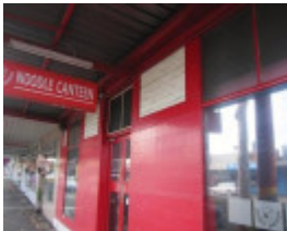
Detail of the west elevation.
