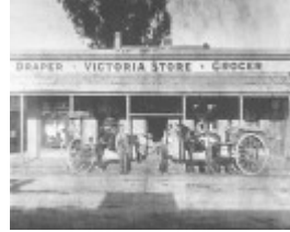
Former 'Victoria Store' pictured in 1902. Note the expansion to the north and south (Source: City of Greater Bendigo).
