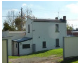
Two storey structure at the rear of the property.
