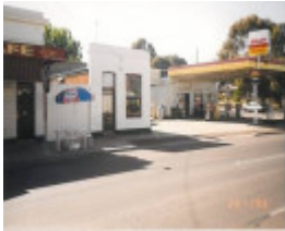
No. 149 High Street (centre) pictured in November 1993. (Source: Andrew Ward, courtesy of City of Greater Bendigo.)
