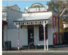
West elevation, addressing High Street, 2010.
