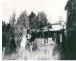
B3226 Parslow's House From Cooper Street
