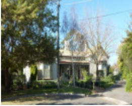
West elevation of Myrnong.
