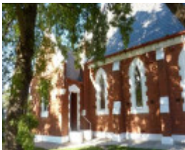
Entry to the sacristy (north elevation).
