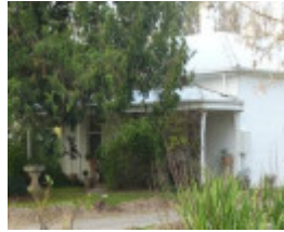
Detail of verandah.
