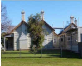
East elevation of the police station and quarters, showing the three 1880s transverse gables.
