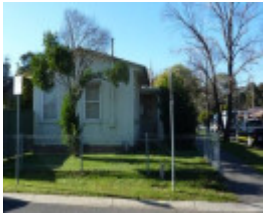
West elevation of the freestanding 1963 addition at the south-west corner of the site.
