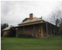
View of Ark Hall looking directly east.
