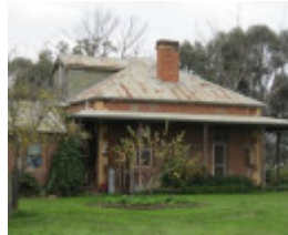
South-east elevation, note timber dormer at rear.
