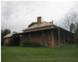
View of Ark Hall looking directly east.
