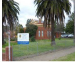
West elevation, note mature palms.
