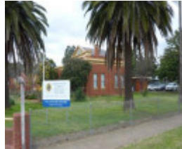
West elevation, note mature palms.
