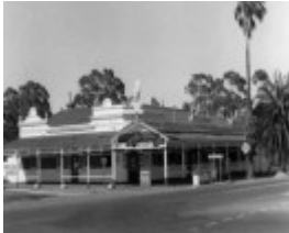
Marong Hotel, looking north-east, 1986 (Source: State Library of Victoria, jc011775).
