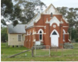
West elevation, with timber addition at rear and bell tower to north of entry.
