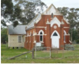
West elevation, with timber addition at rear and bell tower to north of entry.
