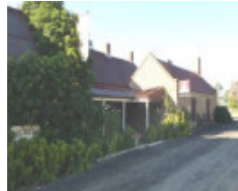
West elevation, with gabled addition at south end (right).
