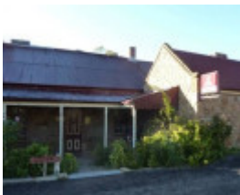
Former residence, to south of 1865 wing.
