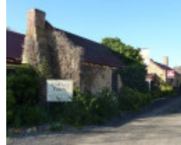
The 1860s wing; note stepped chimney form.
