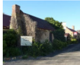
The 1860s wing; note stepped chimney form.
