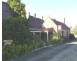
West elevation, with gabled addition at south end (right).
