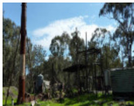
From left, looking north: Metal stack; remnants of brick boiler housing; gantry for truck-mounted vat; and rail carriage (former eucalyptus cutter's hut).
