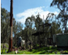
From left, looking north: Metal stack; remnants of brick boiler housing; gantry for truck-mounted vat; and rail carriage (former eucalyptus cutter's hut).
