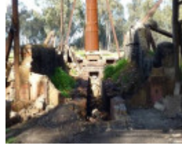
Brick housing for boiler, removed 2010.
