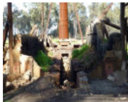
Brick housing for boiler, removed 2010.
