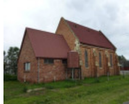
Addition at the rear of the church.
