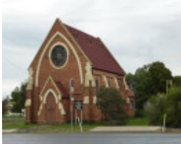
West and north elevations. Note bell tower to the north (right) of the church.
