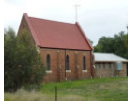
South elevation, note addition to the rear (east).
