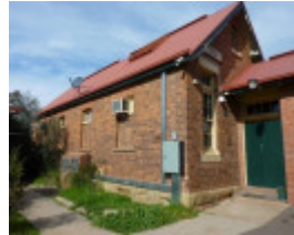
North elevation, note modified windows to school room.
