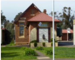
West elevation, with the school room (1877) to the rear of the porch (1912).
