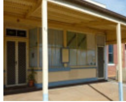
Shopfronts, note two doors and signage ('Confectionary' and 'Soft Drinks') to upper windows.
