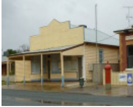
North and west elevations of the former store (pair of shops).
