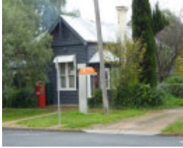
Post office entrance, at east of property.
