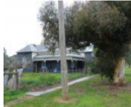
West elevation, as viewed from Inglewood Street.
