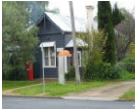
Post office entrance, at east of property.
