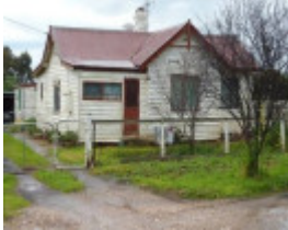
South elevation. Note infilled verandah to the west of the projecting gable.
