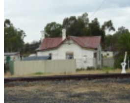
West elevation, with the rail track in the foreground.
