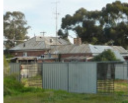
Rear view of the Little Sebastian, as seen from Vogeles Road.
