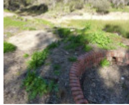
Brick vats adjacent to the stack.
