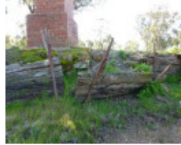
Section of the timber retaining wall.
