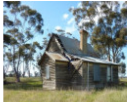
North and west elevations, note sugar gums at rear.
