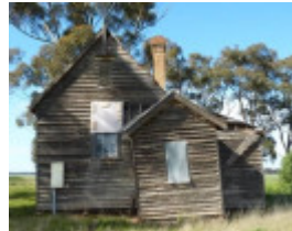
North elevation of the Former Kamarooka Road School.
