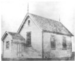
Standard timber school room and porch with capacity for 40 pupils designed in 1872. The picture is not dated, and the school room is not named.
